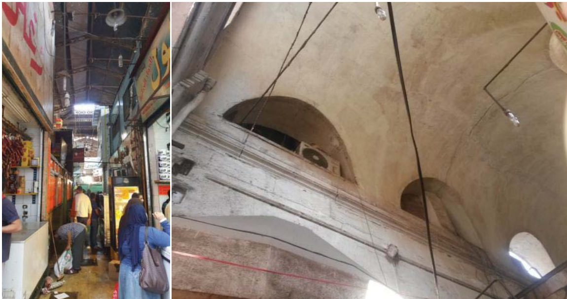
Figure 7. (Left) narrowed alleys (Source: author's collection); (Right) blockage of clerestory windows inside of the building (Source: Authors).
